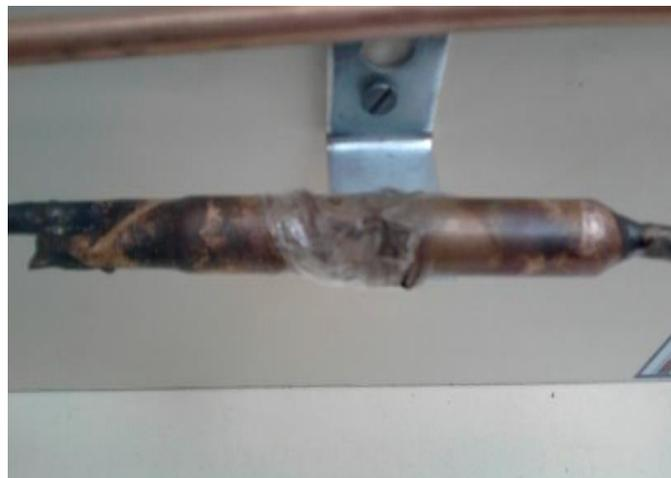
Figure 8: Drier used in VCRS
