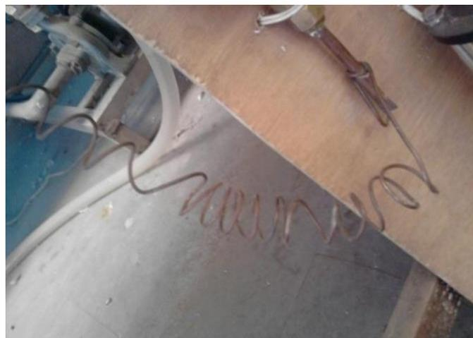
Figure 9: Capillary tube used in VCRS
